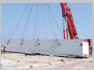
Standard U-Blocks (Dutch floating Breakwaters) 135 tons lifted by crane
