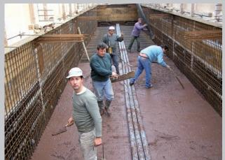
Concrete pouring top wall Dutch Floating breakwater elements
